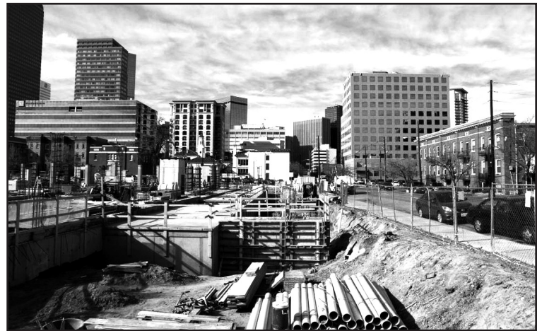
A construction shot of One City Block shows skyline views.
