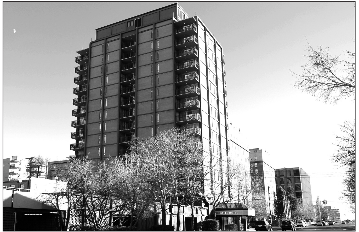
RedPeak Properties plans to turn the Burnsley Hotel into a Class A apartment community.
